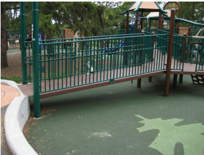
Diagram 48.A Example of accessible entry/exist point and accessible route leading to elevate play components.
