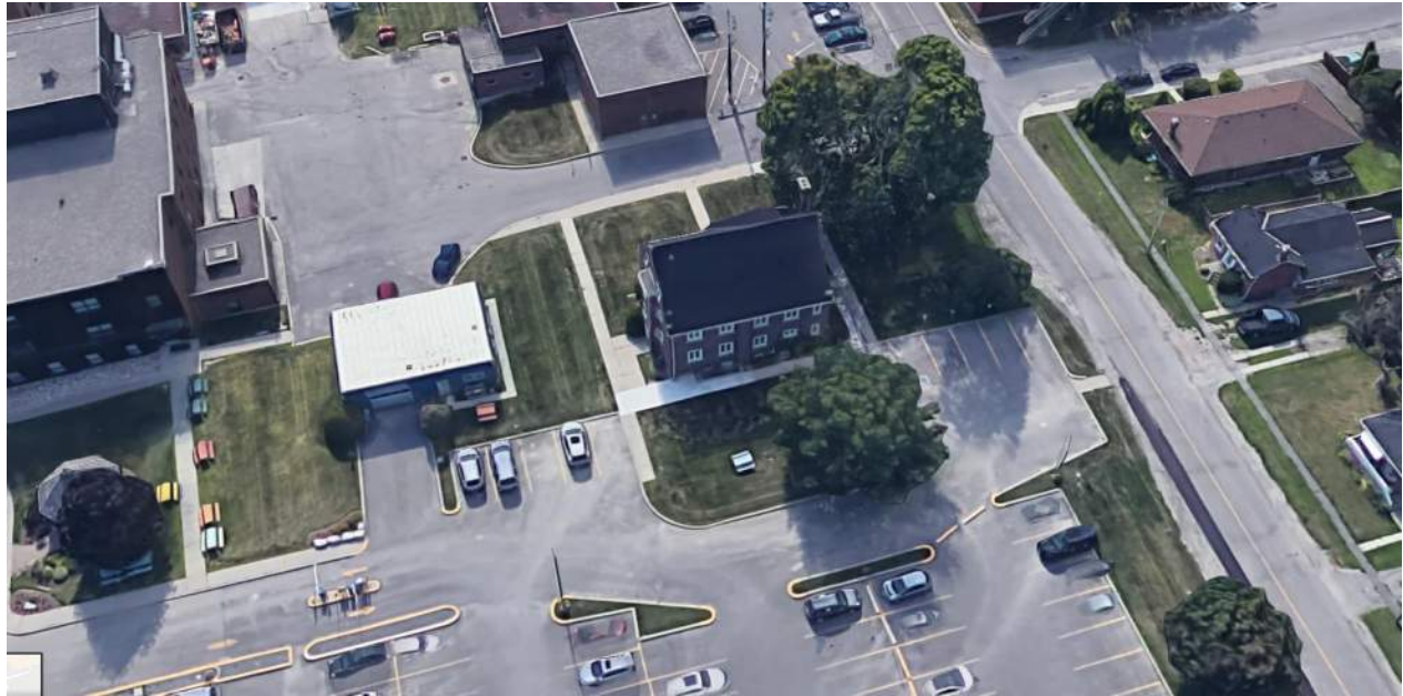
4.1.5.C – Aerial View from East (note: tree along Queen St. frontage has been removed.)
