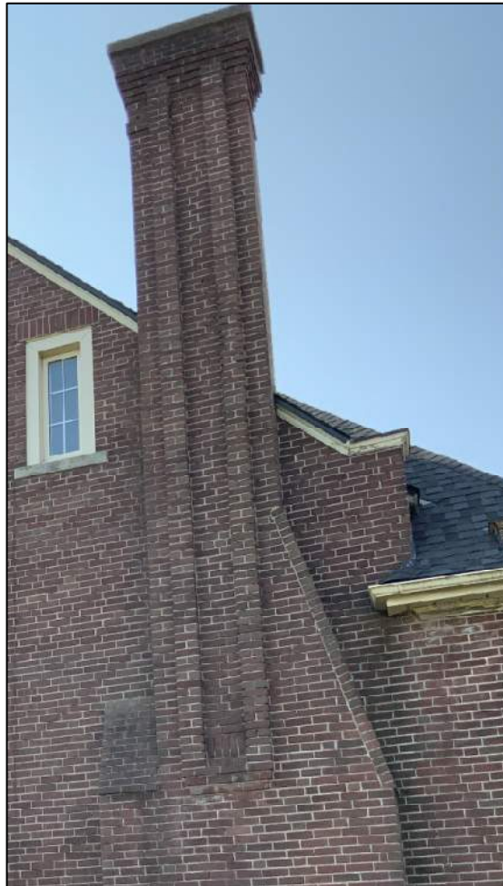
Photograph 6: Chimney, north elevation
