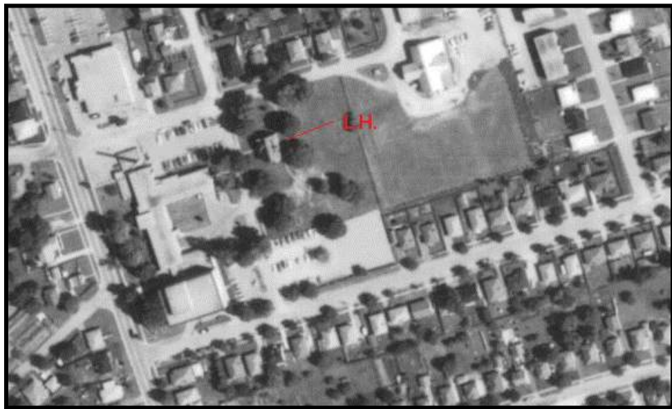
4.2.4.E - Hospital 1971 – South Wing addition
