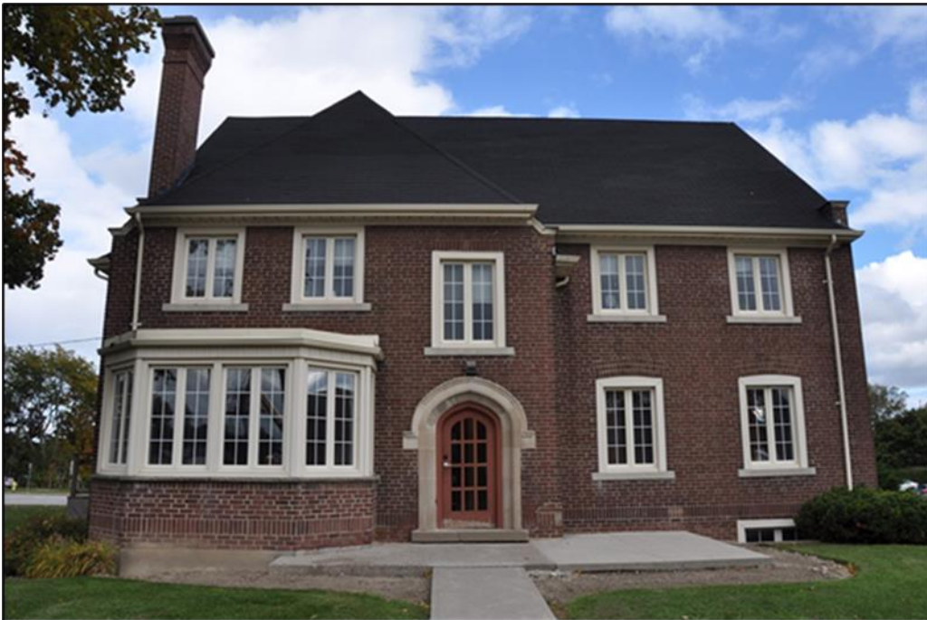
Figure 3: View of the Lambert House from Maple Bruce Way
