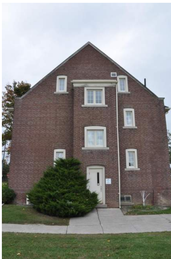
4.1.5.1.B – Existing South (Right) Elevation
