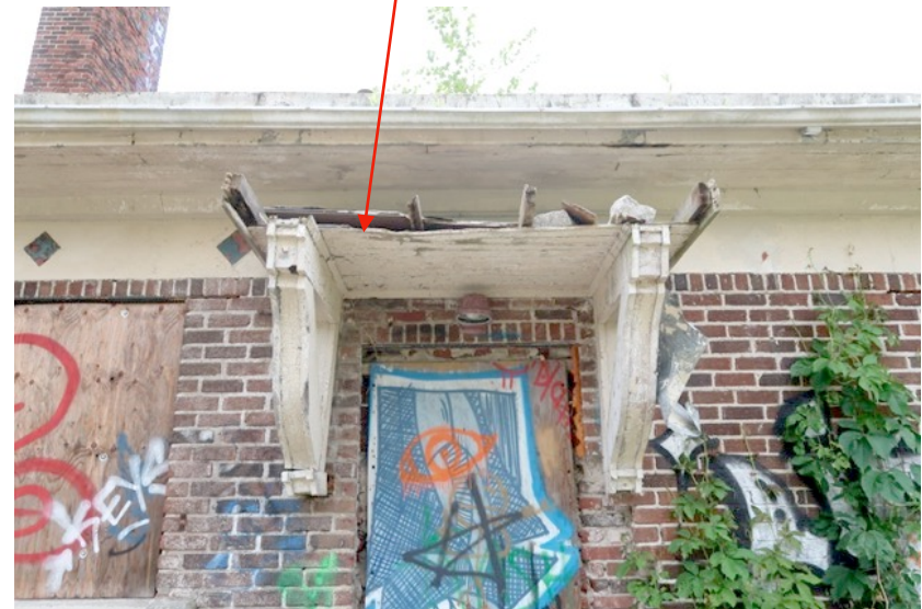
Remains of Canopy roof facing north.
