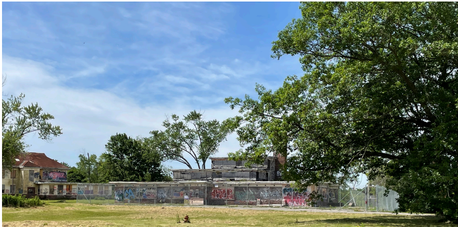
Cafeteria building, east side, July 2024
