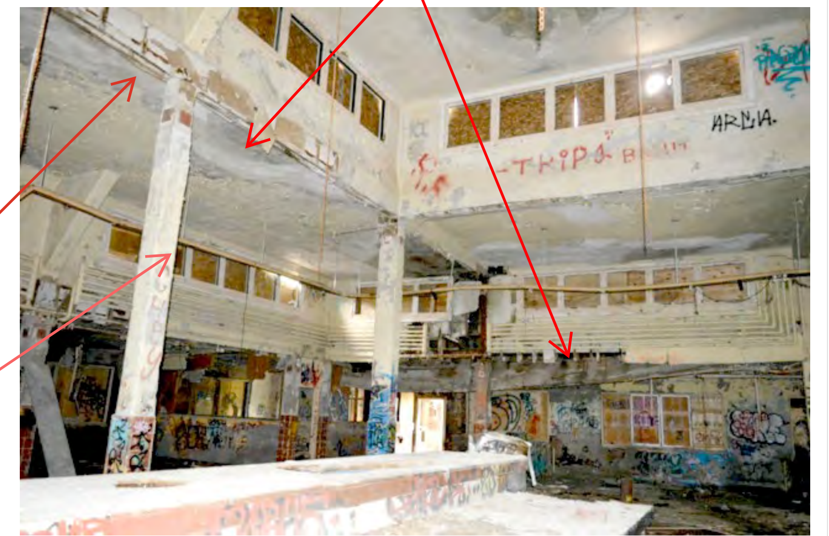
B INTERIOR LOOKING SOUTH WEST
