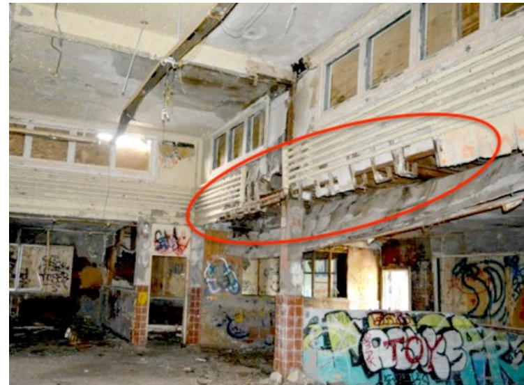
Corresponding interior view of south wall showing deterioration of wall and ceiling at the first tier.
