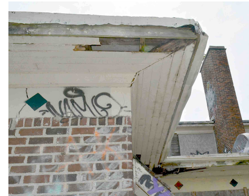
Wood Soffit, Fascia Board & Cove moulding
