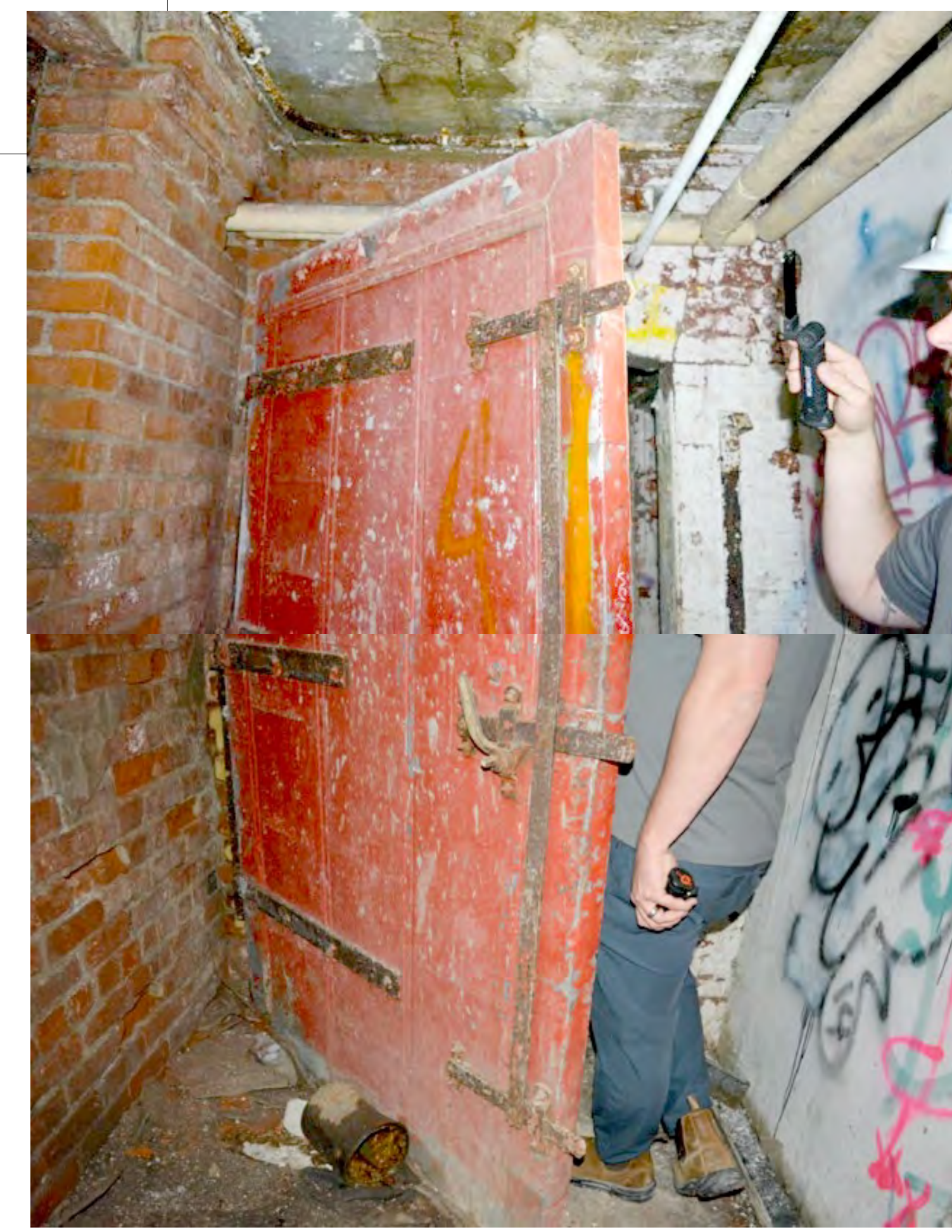
BASEMENT BOILER ROOM DOOR
