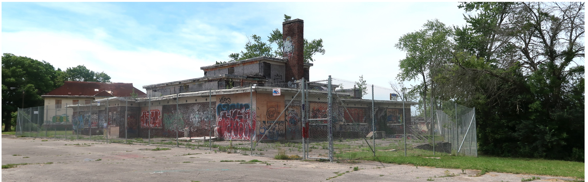
Cafeteria building, south east side, July 2024
