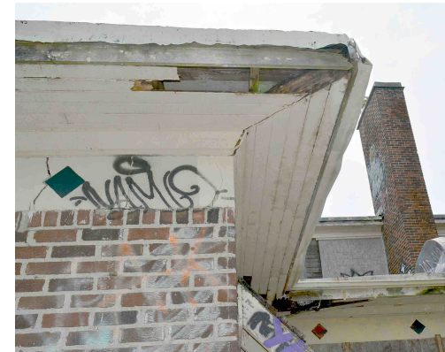
Wood Soffit, Fascia Board & Cove moulding
