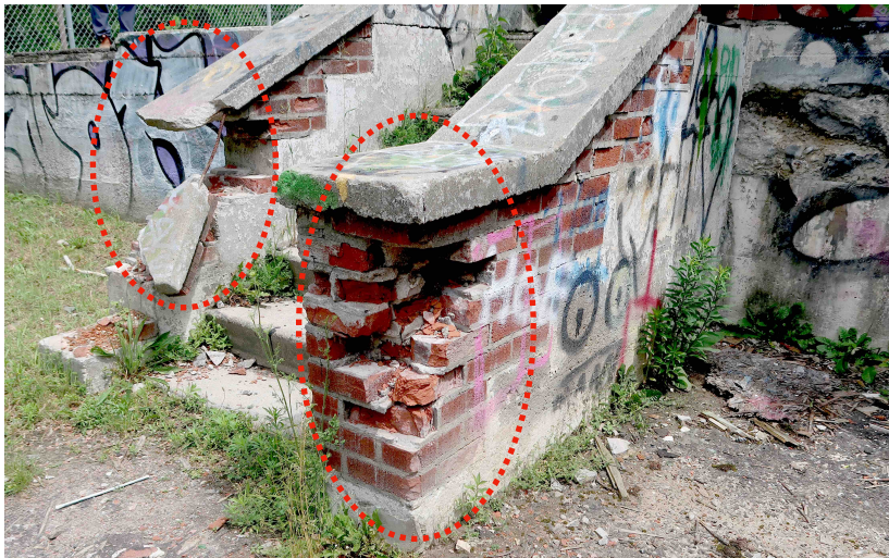
Steps on north side extensively deteriorated and may have been subjected to vandalism
