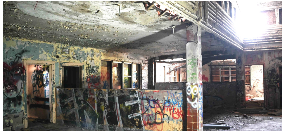
Cafeteria building, interior photograph, July 2024
