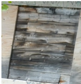
Corresponding interior view of south wall showing deterioration of wall and ceiling at the first tier.
