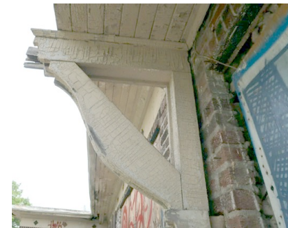
Wood Soffit, Fascia Board & Cove moulding
