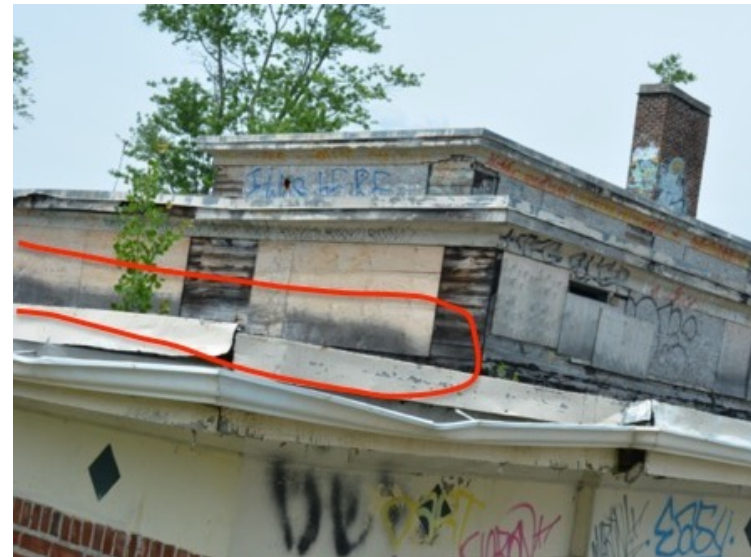
Exterior view of south wall showing evidence of water accumulation at the first tier clerestory level.
