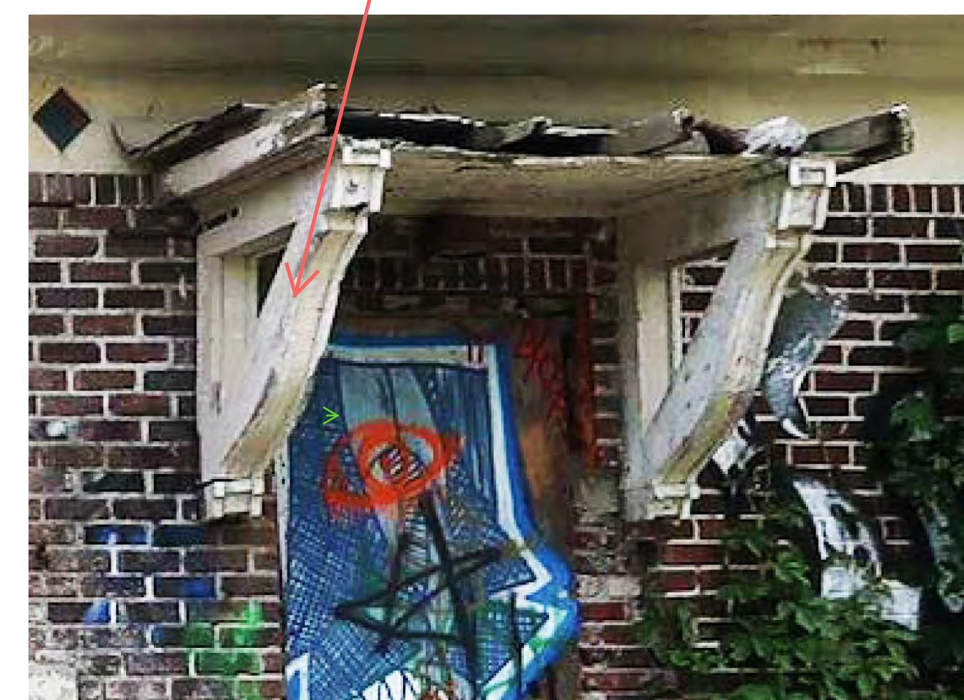
DETERIORATED CANOPY
