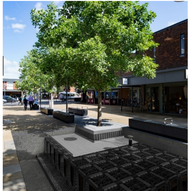
Figure 39: Soil cells can provide the required soil volume for street trees in urbanized areas
