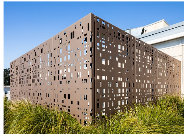
Figure 22: Screen rooftop equipment and utilities from the public view
