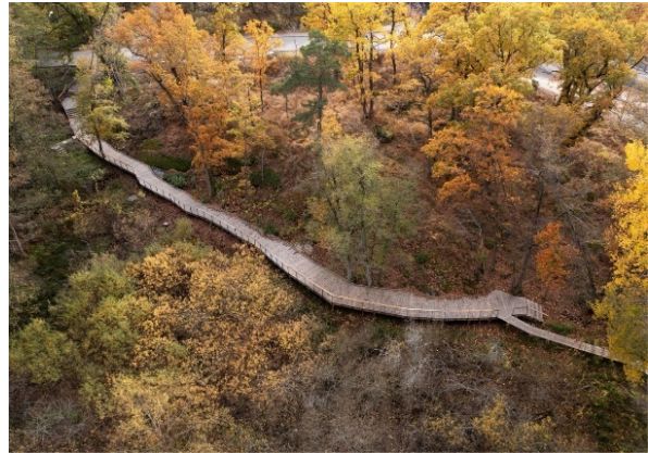
Figure 36: Consider the inclusion of boardwalks in EPAs
