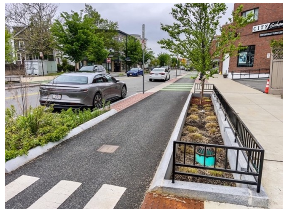
Figure 48: Bioswales help to collect runoff after storm events
