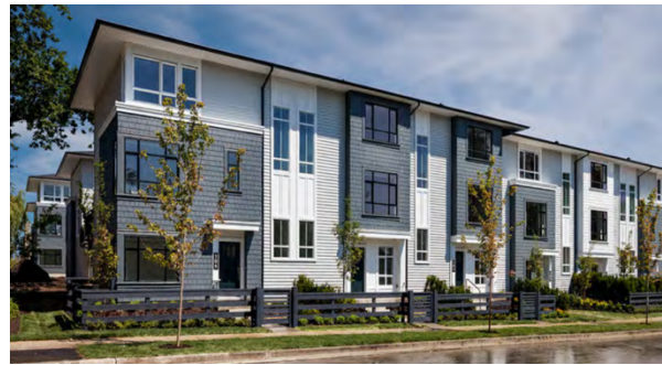
Figure 14: Example of a rear-lane townhouse
