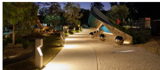
Figure 55: Choose light fixture that are Dark Sky Compliant that direct light down to minimize light spillage onto other properties
