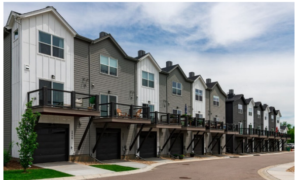
Figure 16: Example of a rear-lane townhouse
