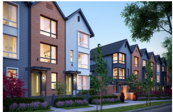
Figure 9: Example of townhouses with high-quality architectural detail
