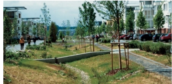
Figure 50: Example of a Bioswale
