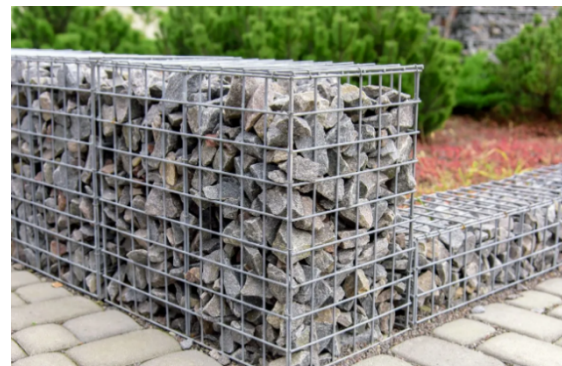
Figure 52: Reclaimed materials can be used for new infrastructure such as gabion walls
