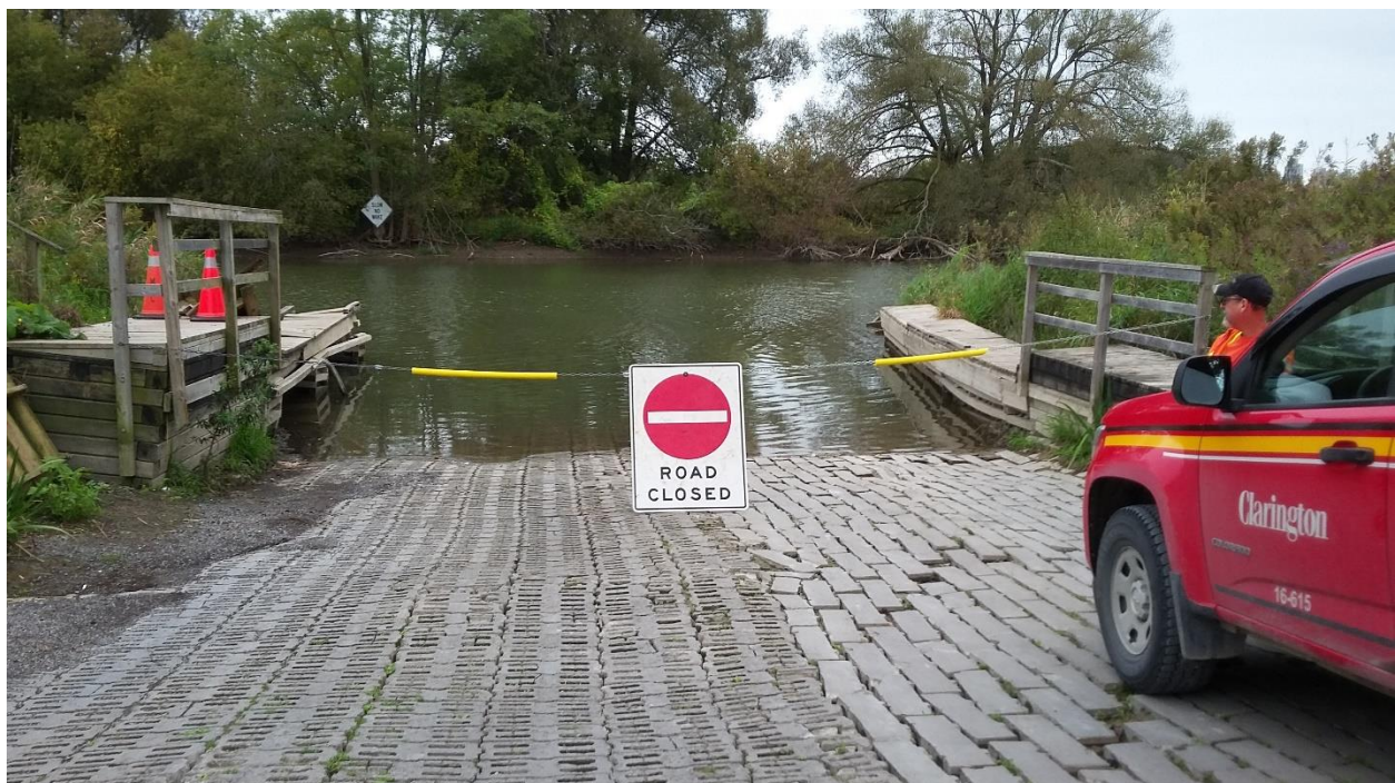
Figure 4: Bowmanville Boat Launch Ramp
