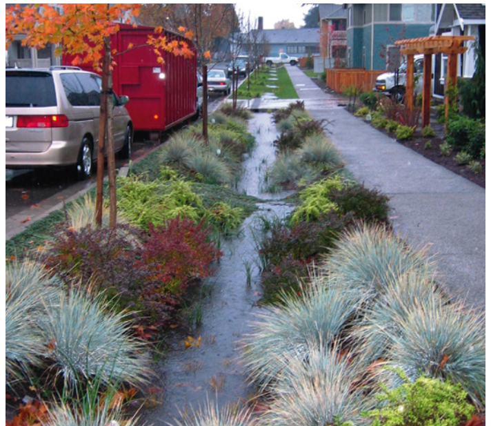
Low-impact development, such as rain gardens and bio-swales, should be considered wherever possible to complement the stormwater management strategy
