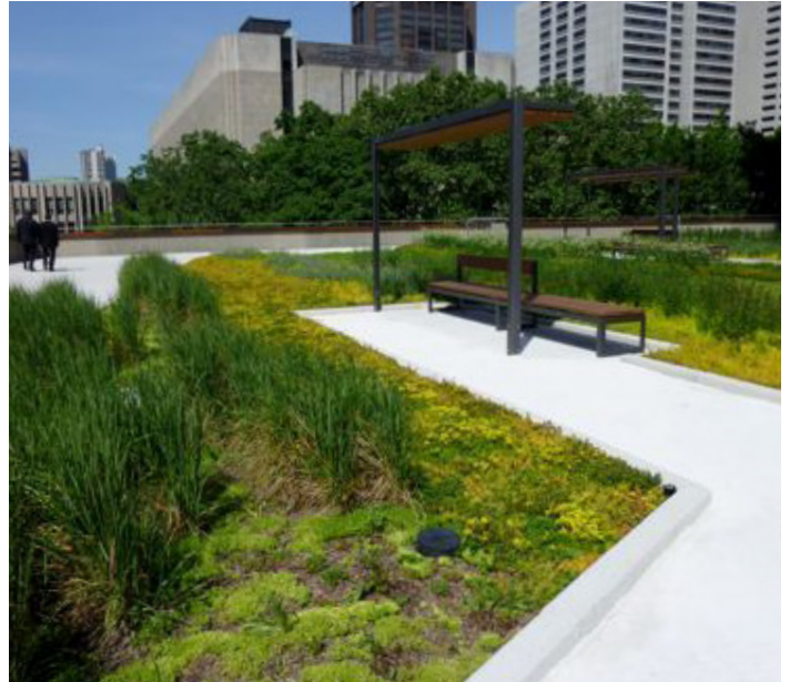
Green roofs can have several benefits such as water retention and treatment, insulation, habitat and private amenity space.
