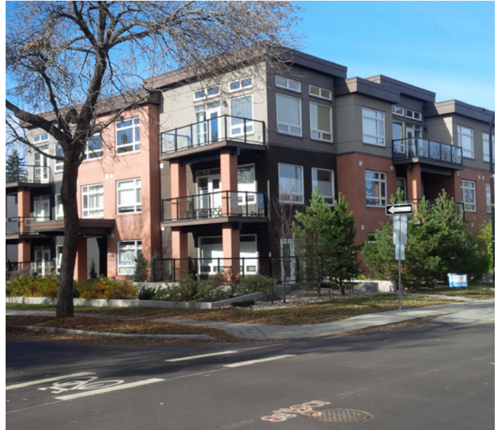
Low-rise apartment buildings up to 4 storeys provide an opportunity for more activity along arterial roads
