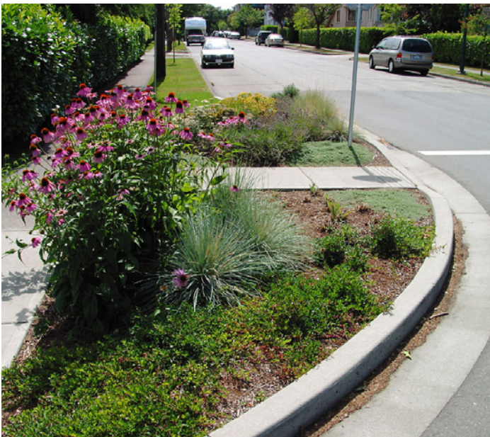
Well designed and landscaped curb extensions permit on-street parking and safe pedestrian crossings to coexist
