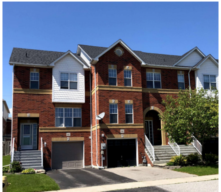
Example of existing townhouses in Bayview
