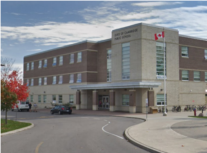
The front entrance of the school is accentuated with architectural features and detailing, and is connected with a walkway.
