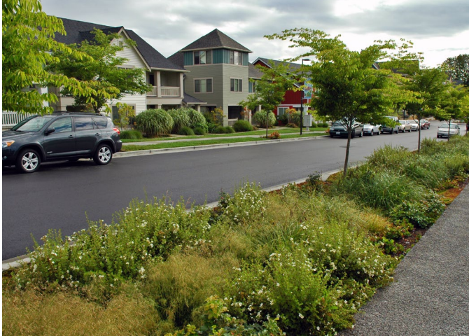
Bioswales in the public right of way to improve infiltration.
