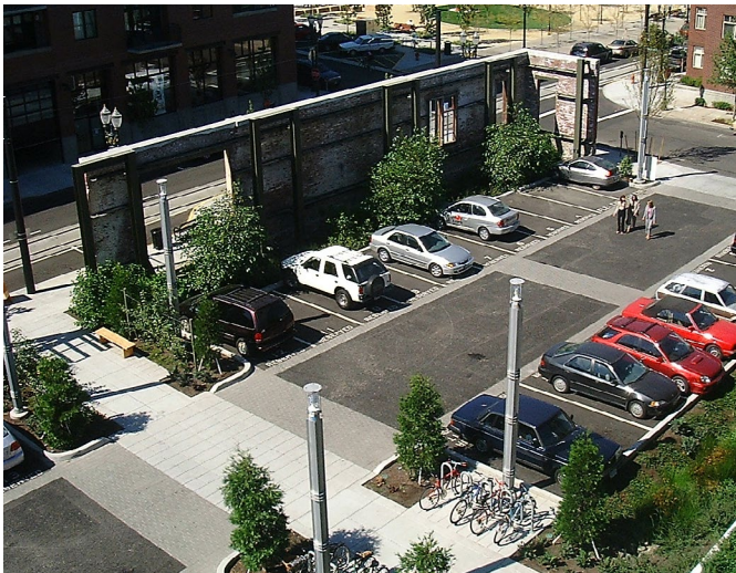
Parking lot with smaller courts, plantings, and decorative paving.
