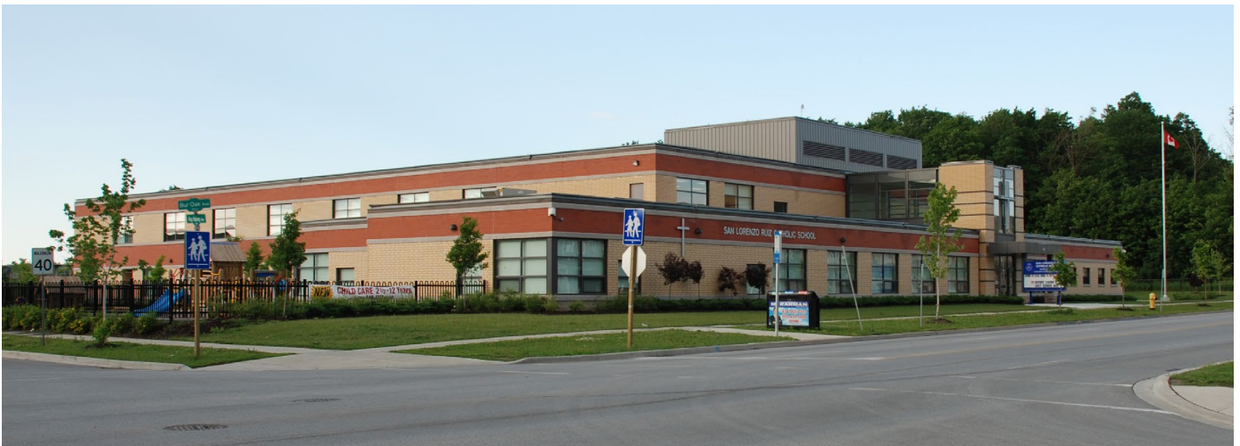
Parking is located to the rear of the building off the main road and the front entrance to the building is directly connected to the public sidewalk.
