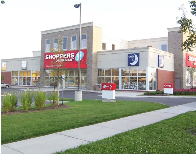
Example of a commercial building.
