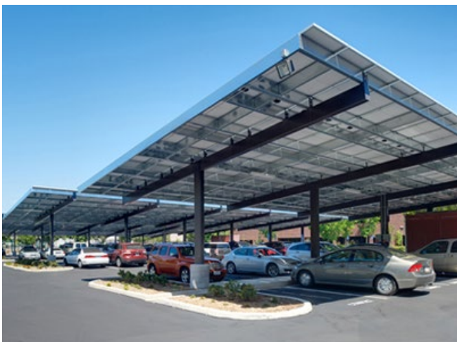
Solar canopies in surface parking lots.
