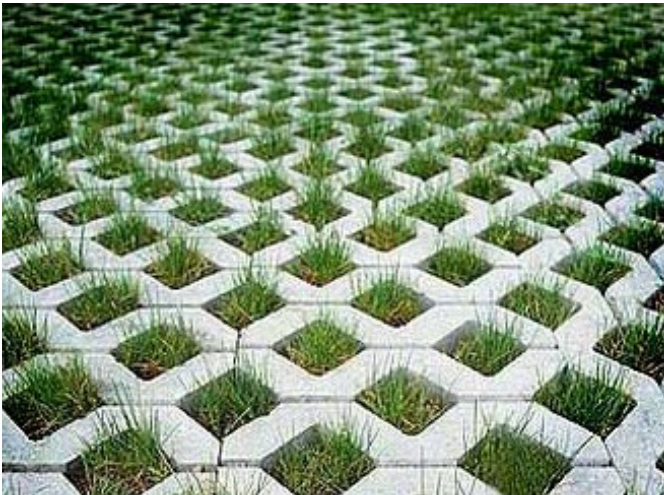
Permeable pavers to support on-site stormwater infiltration.
