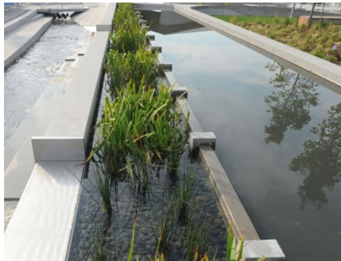
Innovative stormwater management facility.
