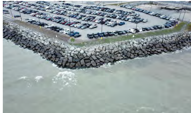
Shore Protection fronting Darlington Nuclear Power Plant
