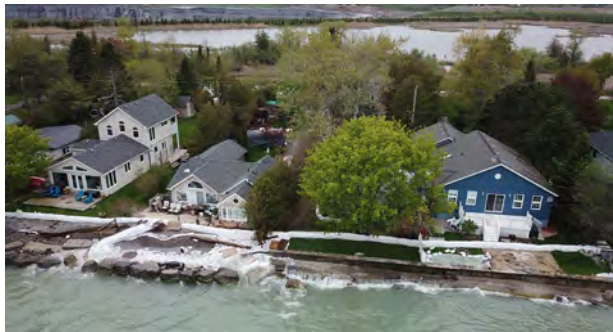
Cedar Crest Beach Blvd. during Record High Water Levels (May 2019)
