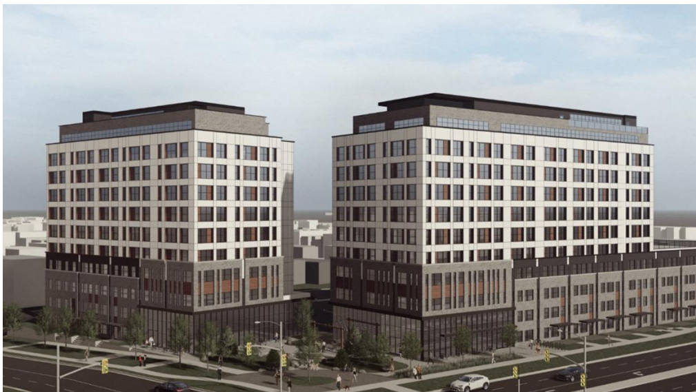
Figure 3: South-east perspective of the proposed 11 storey buildings
