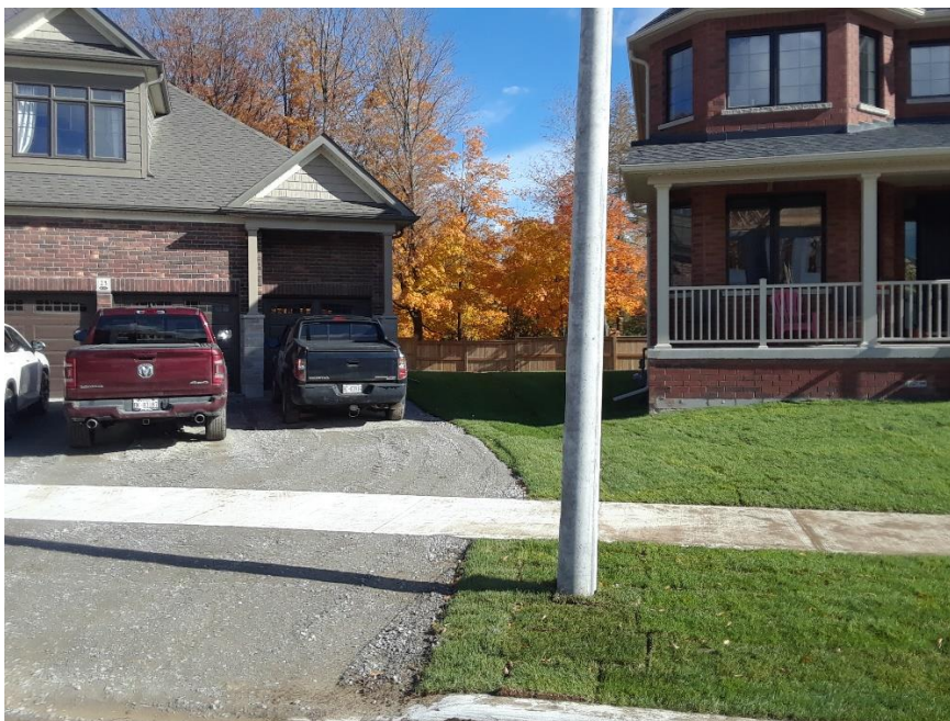
Figure 1: Photo of streetlight at 23 Harry Lee Crescent
