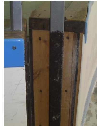
Figure 13: Signs of metal rusting at door interfaces.
