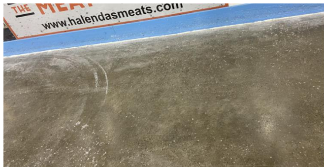
Figure 10: Large scrapes found on the rink floor
