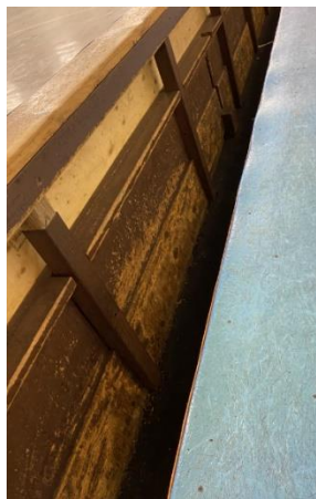
Figure 12: Scuffing and wood damage near foot level.
