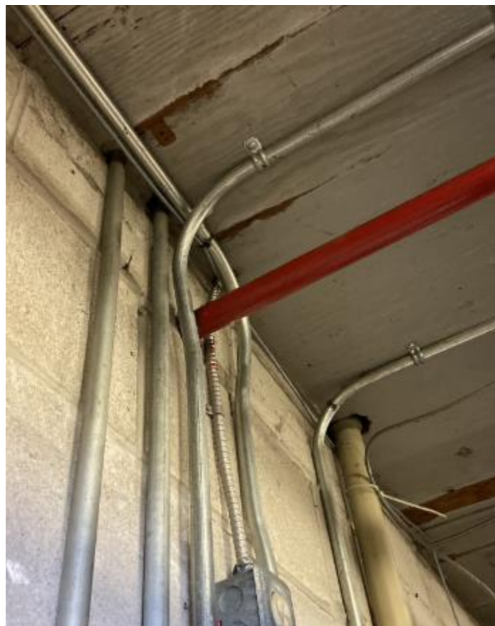
6.3 f) Pipes passing through walls and ceiling not properly sealed
