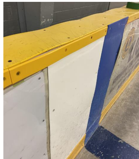
Figure 13: Waviness in board facings
