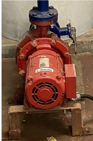
Figure 6: Condenser Pump
