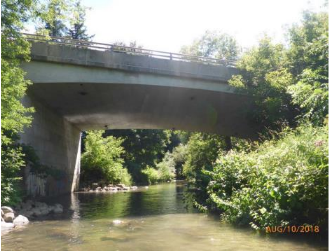
King Street East Bridge (Bowmanville, On)
