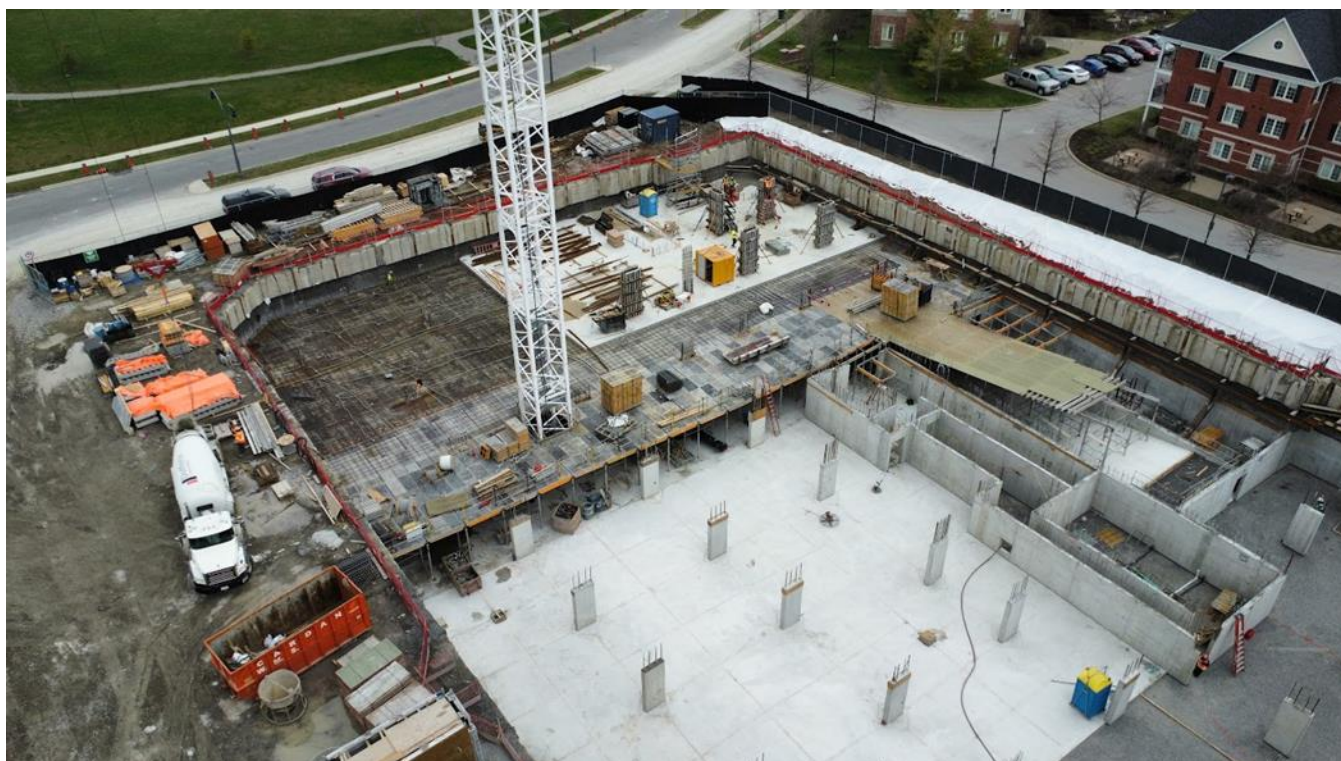
Figure 2: Drone Imagery from April 2023 of 55 Clarington Boulevard (Construction on Underground Parking)
