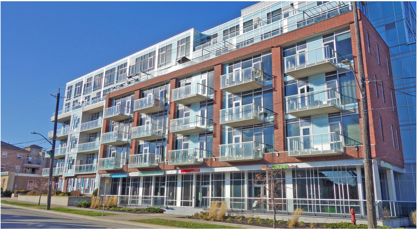
Figure 17: This building has a 4 storey podium. Above the podium the building is stepped back. This is appropriate for the Downtown Corridor, East Business District and Goodyear Lands Character Areas.
