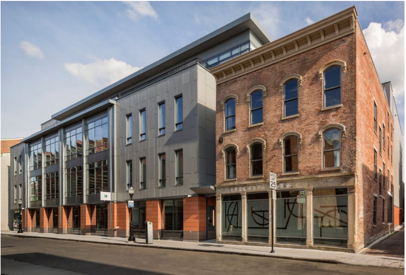
Figure 18: In the Historic Downtown Character Area, podiums should be 2 to 3 storeys in height to match the existing context. Above the podium the building is stepped back.
