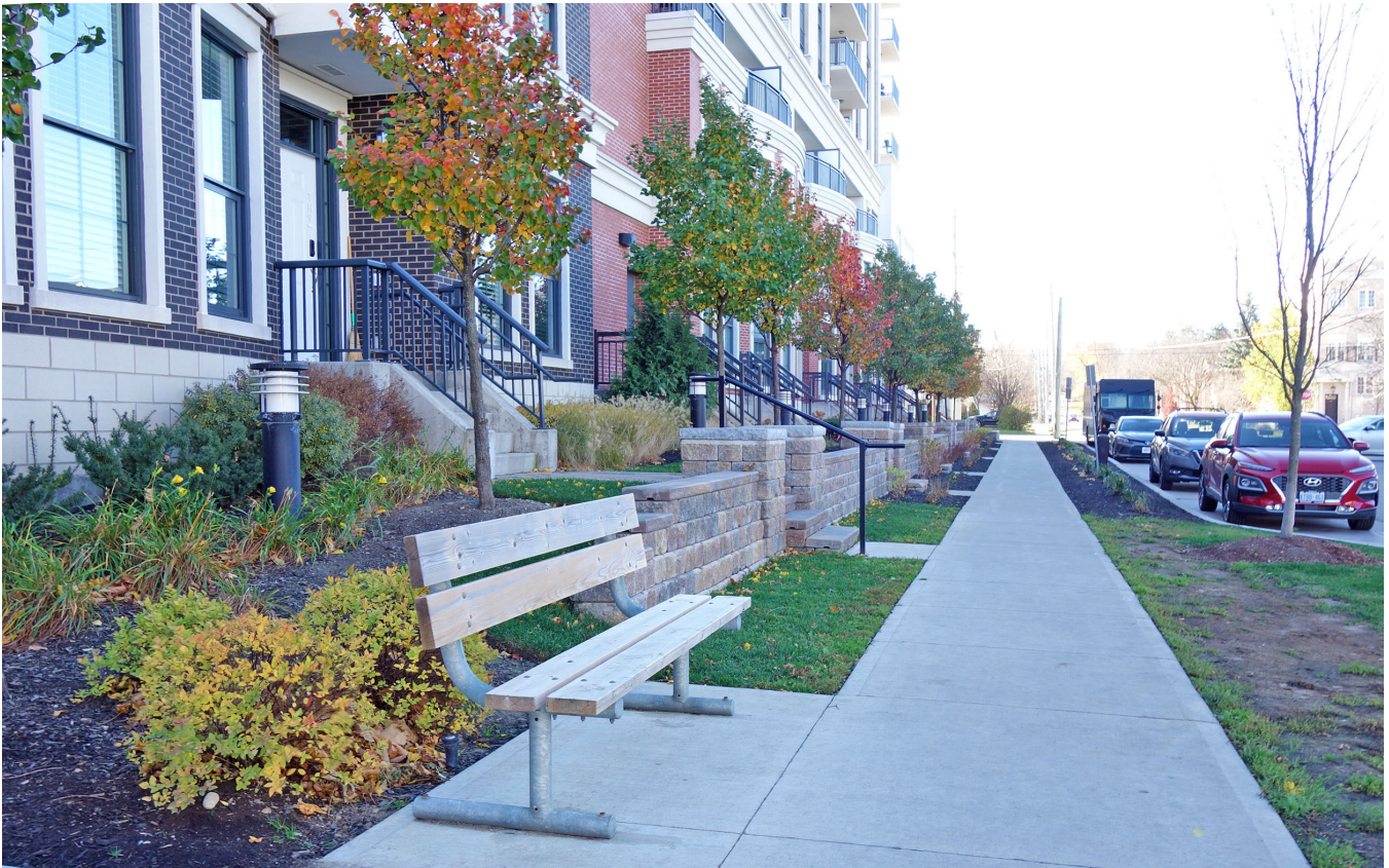
Figure 14: Ground level units are individually articulated in the architectural expression. Each has a direct entrance to the adjacent sidewalk with a small front yard transition zone.
