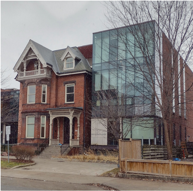
Figure 42: New development references datum lines in the heritage building, including roof lines, eave lines, and vertical proportions. The new development creates a sense of separation and distinctness from the heritage building through a recess (shadow line) where it is joined, and by using a distinctly different material (glass).
