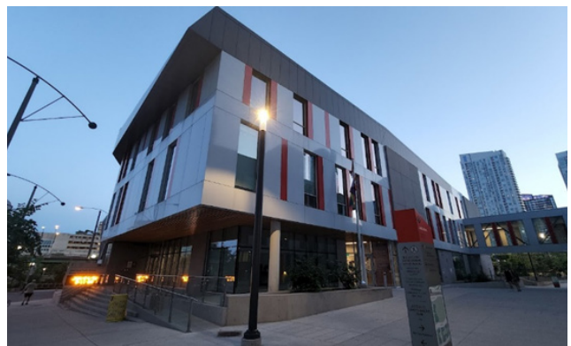
Figure 41: Urban-scaled mixed-use schools. Precedents: Crosstown Elementary School in Vancouver and Jean Lumb Public School / Canoe Landing Community Centre in Toronto
