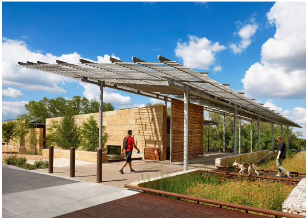
Washroom building with a shade canopy
