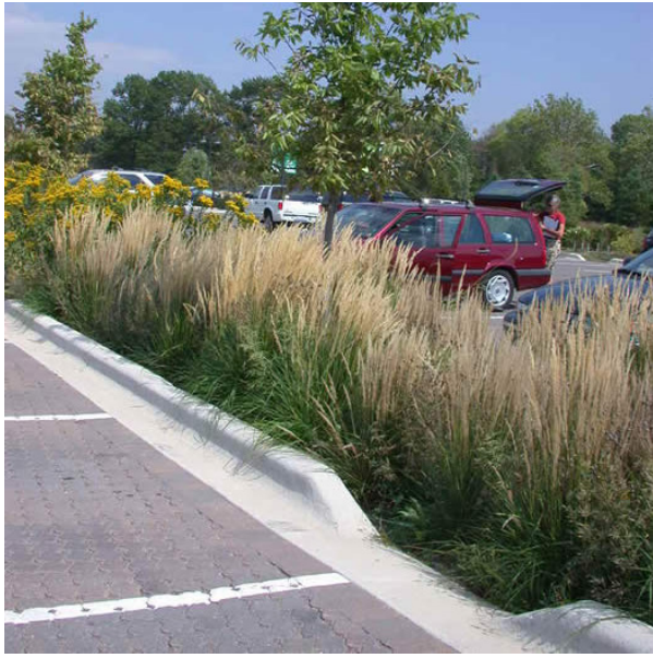
Permeable Pavers in Parking Area
