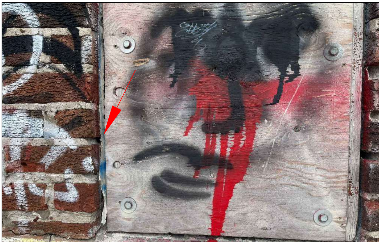
Photograph 12 Asbestos Containing on Window Caulking on Exterior South Wall
