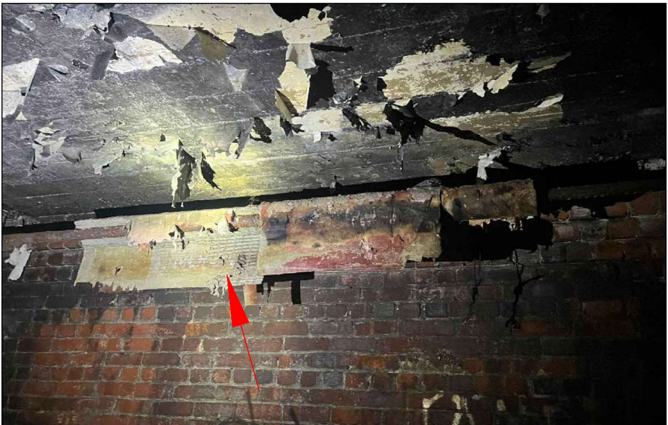
Photograph 4 Air-Cell and Parging Cement Insulation in South East Basement Room
