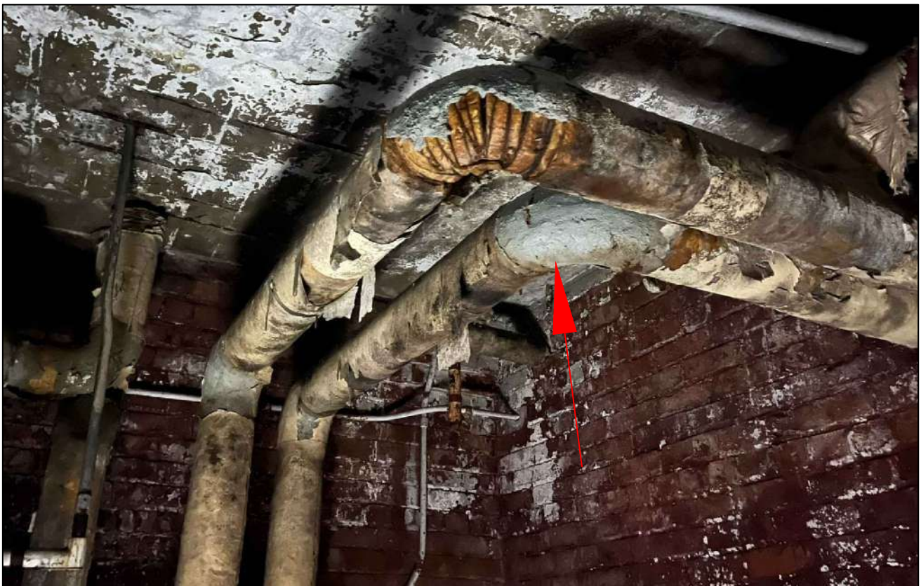
Photograph 6 Parging Cement Insulation on Pipe Elbow in Boiler Room
