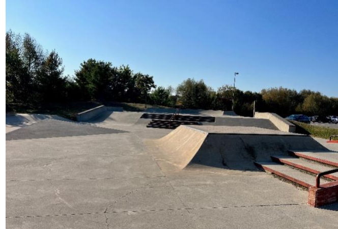
Courtice Community Complex
