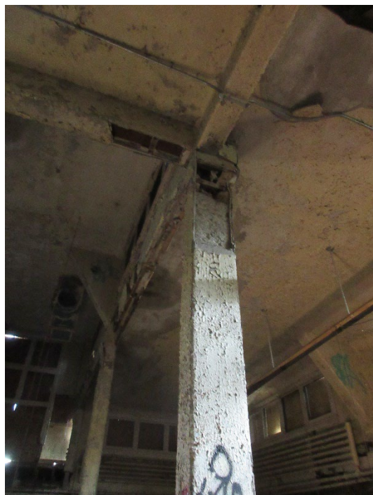
Photo 007 – Ground Floor Concrete Encased Beams and Columns
