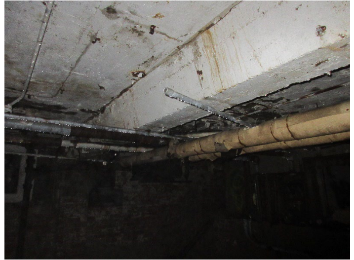
Photo 014 – Concrete Encased Beam
