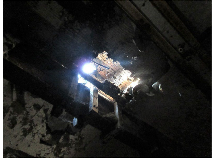
Photo 002 – Rotted Decking Viewed from below
