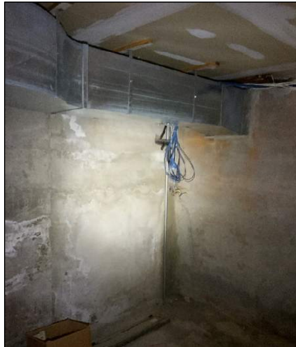
Photograph 2: Exterior foundation wall (typical)
