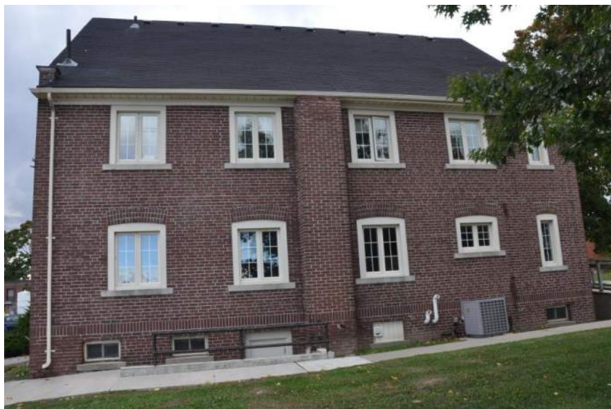
4.1.5.1.C – Existing East (Rear) Elevation
