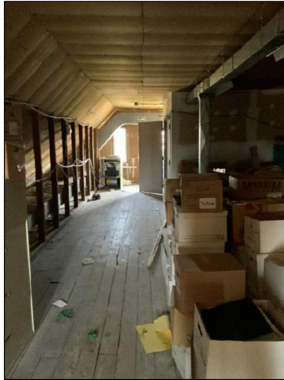
Photograph 1: Attic space (typical)
