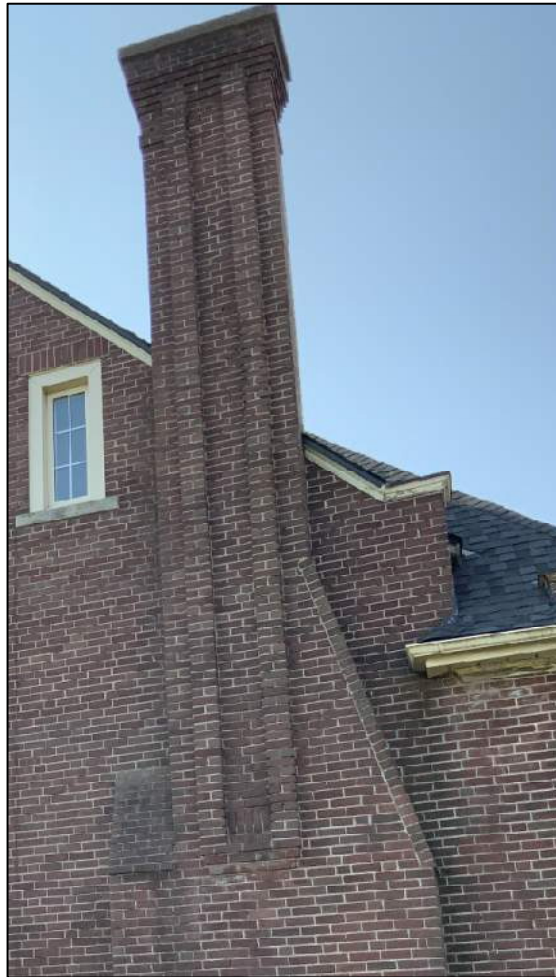
Photograph 6: Chimney, north elevation
