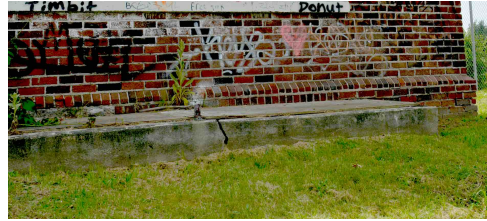
Crack in north window well.
