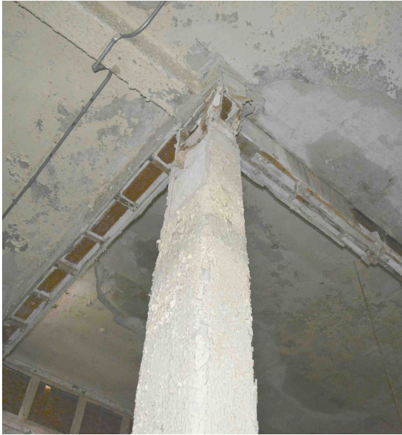
Steel Column encased in clay tile and parging.
