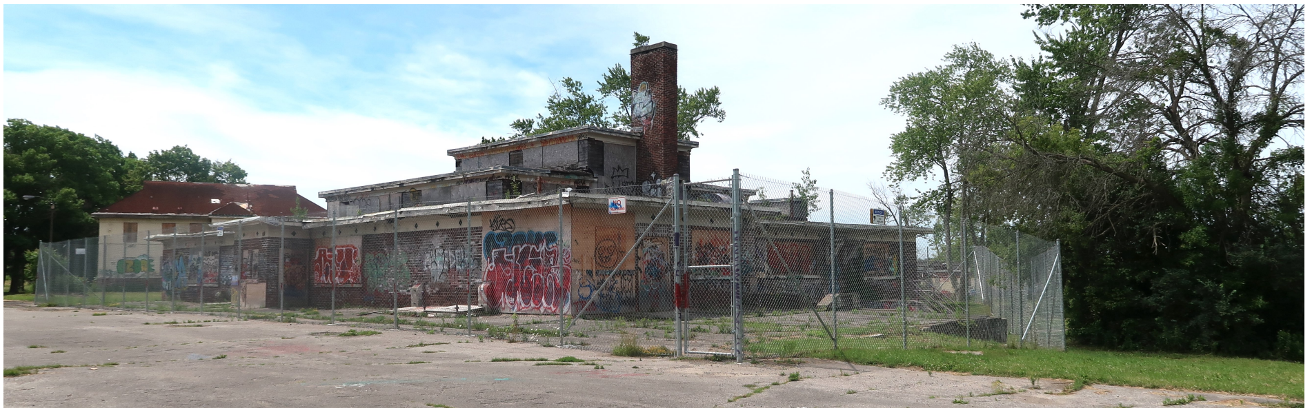
Cafeteria building, south east side, July 2024
