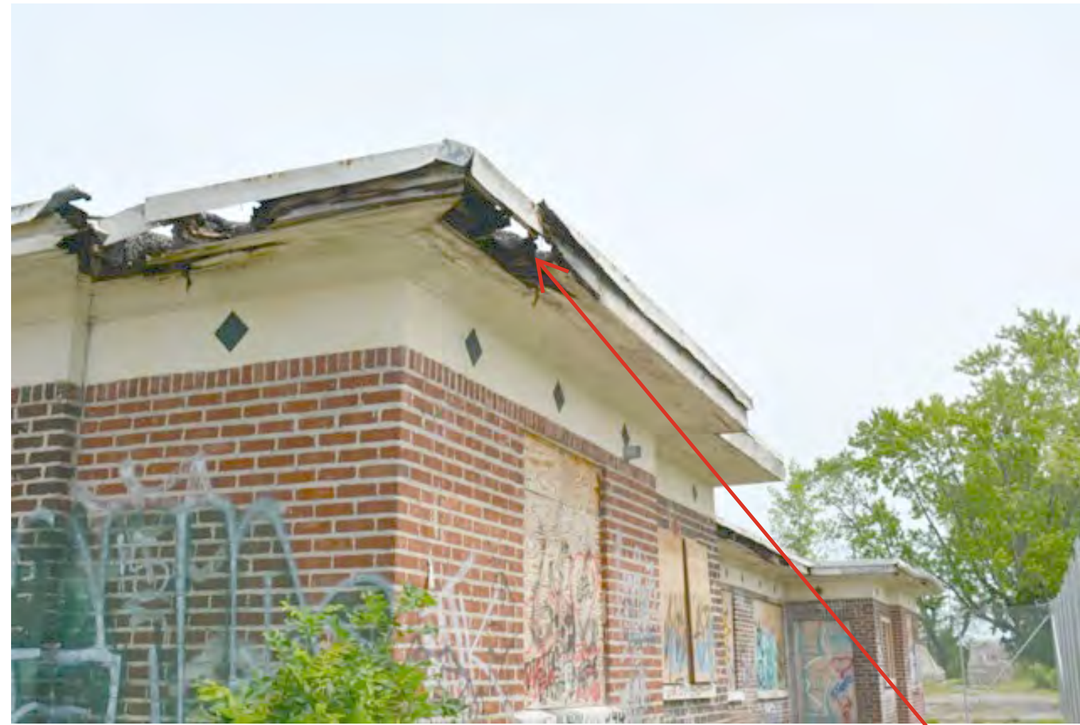
ROOF STRUCTURE HEAVILY DETERIORATED AT EDGE. FASCIA AND SOFFIT SEVERELY DETERIORATED AND DAMAGED. NO GUTTERS
