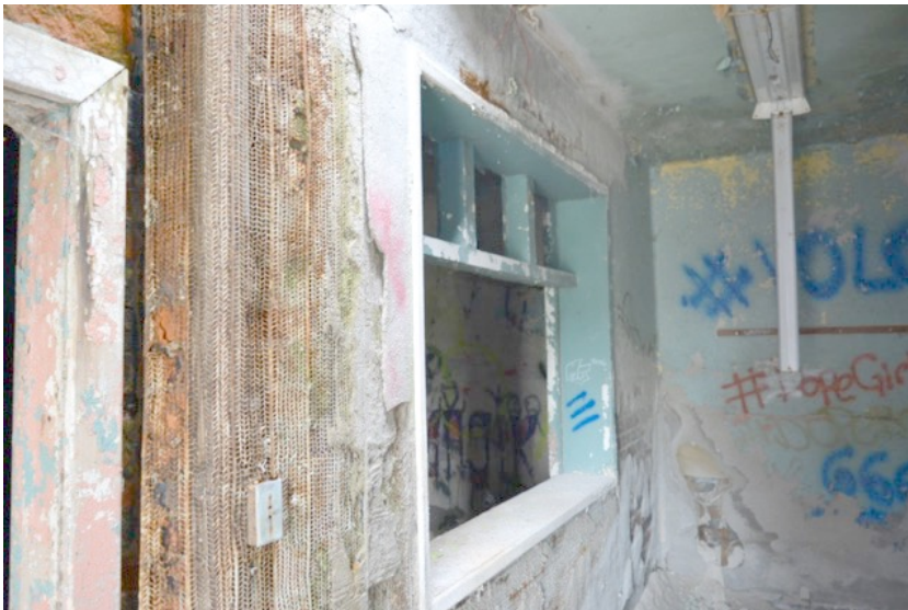
Wood window frame inside south-east addition.
