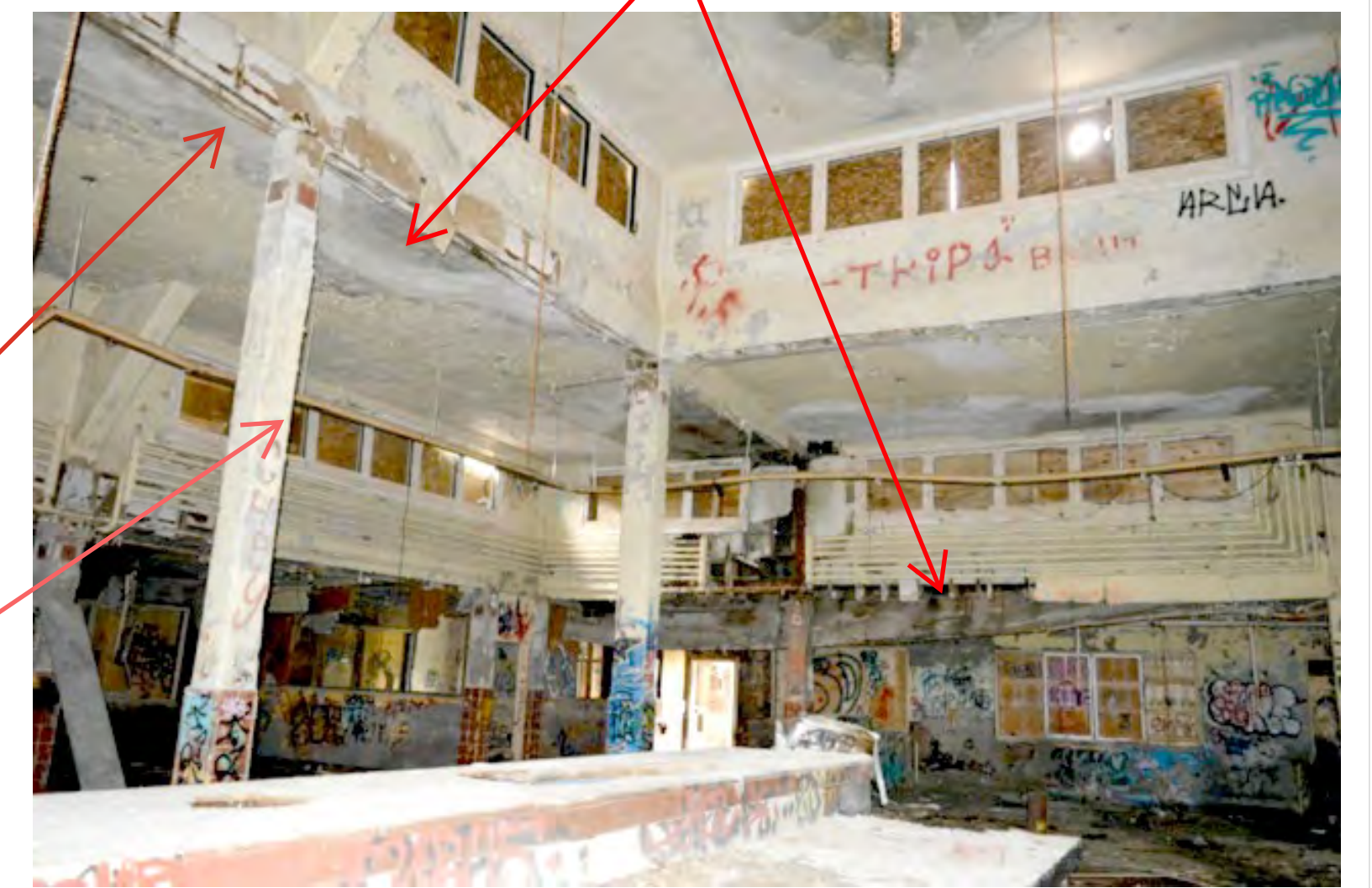
B INTERIOR LOOKING SOUTH WEST
