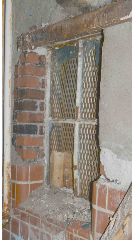
Metal basement window with metal barrier and typically sloped sill.
