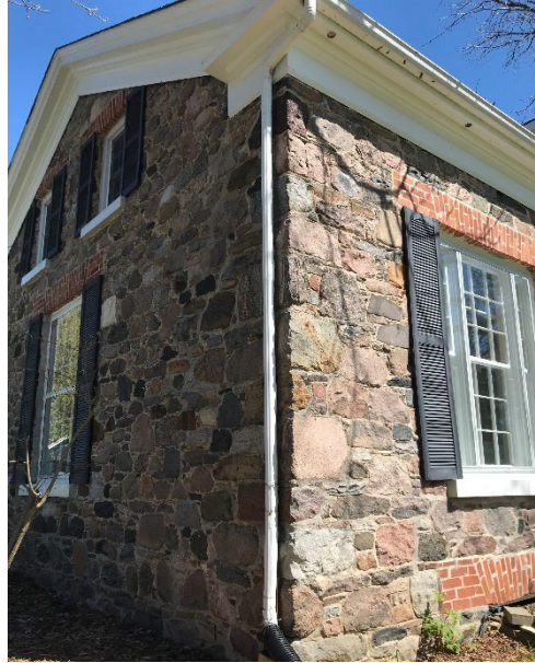
Figure 11: Southwest corner showing "boulder quoins". (May 2024)
