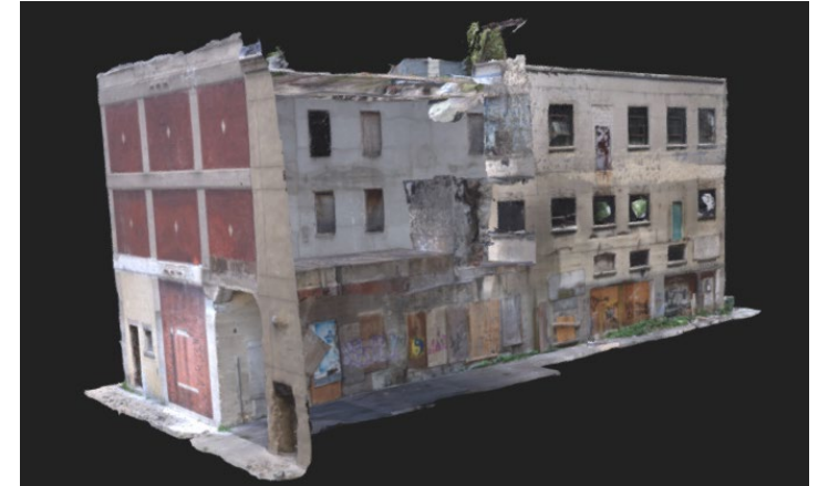
123 Queens Exterior (Stantec 2019)
