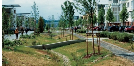
Figure 50: Example of a Bioswale
