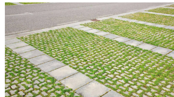
Figure 49: Example of a porous pavement that contributes to runoff management
