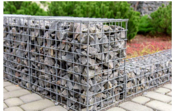
Figure 52: Reclaimed materials can be used for new infrastructure such as gabion walls
